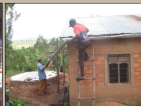
Attaching gutters
